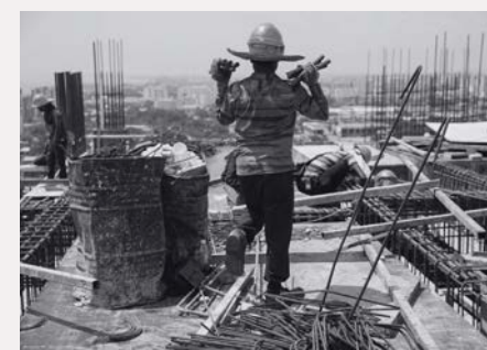
Page: 22 Copyright: Arnaud Finistre Description: Rohingya workers employed on a construction site in Penang. Around half of the workers on the site are Rohingya, who, with no legal status in Malaysia, are not legally allowed to work. The other workers are Bangladeshi, Indian, Indonesian or Malaysian. Rohingya workers often work in particularly precarious safety conditions, frequently sleeping on site in basic shelters to save money. This allows them to send money to their families who have stayed in Myanmar or who have fled to Bangladesh. Some unscrupulous employers take advantage of their irregular legal status to deprive them of their full wages. Construction sites, which are numerous in Malaysia, are one of the few ways the Rohingya can earn a living in the informal economy, but many workers have been cheated out of their earnings. Penang
